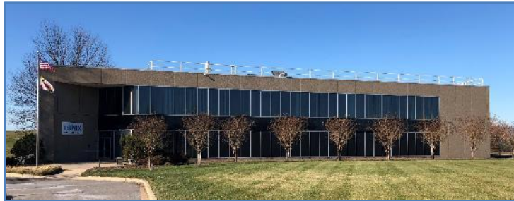
R&D Center- Maryland Operational BSL-3
